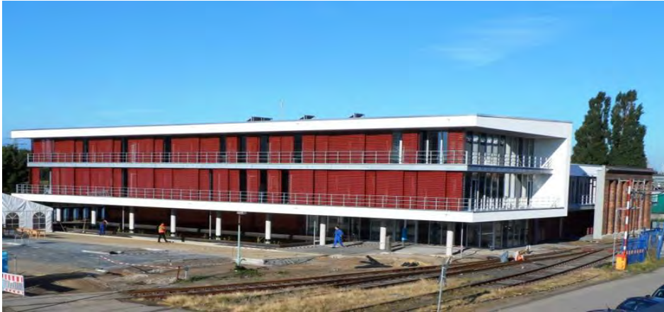
Office port railway (Photo: HPA)
